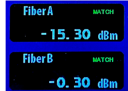
Example display of high attenuation in Fiber A.
